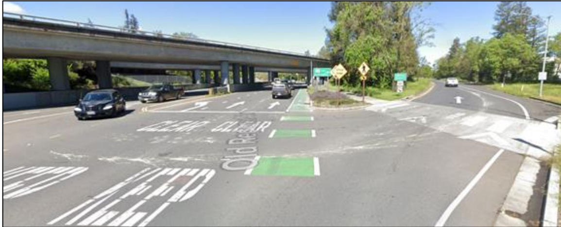
Figure 15. Image showing the Highway 101 underpass at Old Redwood Highway. Note combination of dedicated bike lane, but also freeway on and off ramps that can create unsafe conditions for pedestrians and cyclists, making it less likely for them to use these crossings and limit East/West access across town. Source: Google Street View
